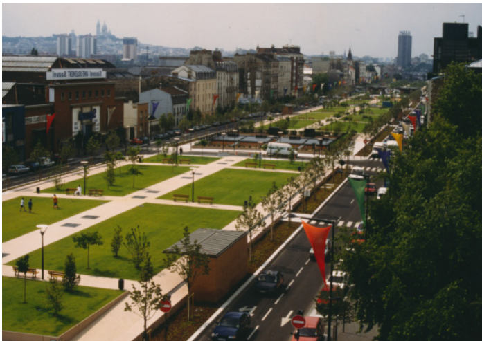
REF: Couverture de l'autoroute A1, Paris, France
